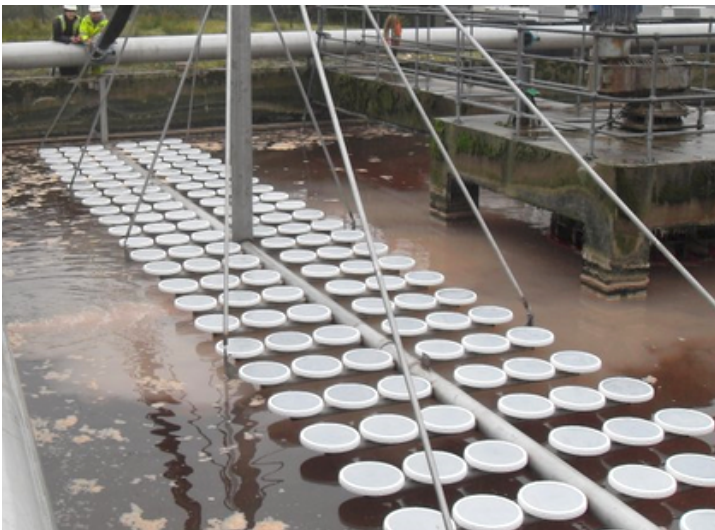
Systems extractable by crane with disc diffusers (on the left) and tubes (on the right)
