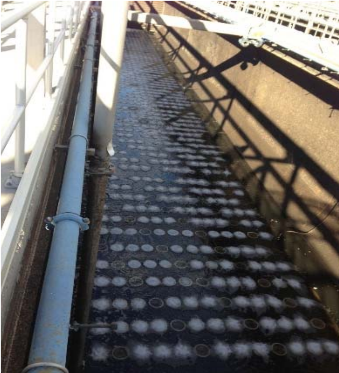
Figure 1: SSI Membrane Diffusers installed in Pass C of Aeration Tank at Bowery Bay Wastewater Treatment Plant
