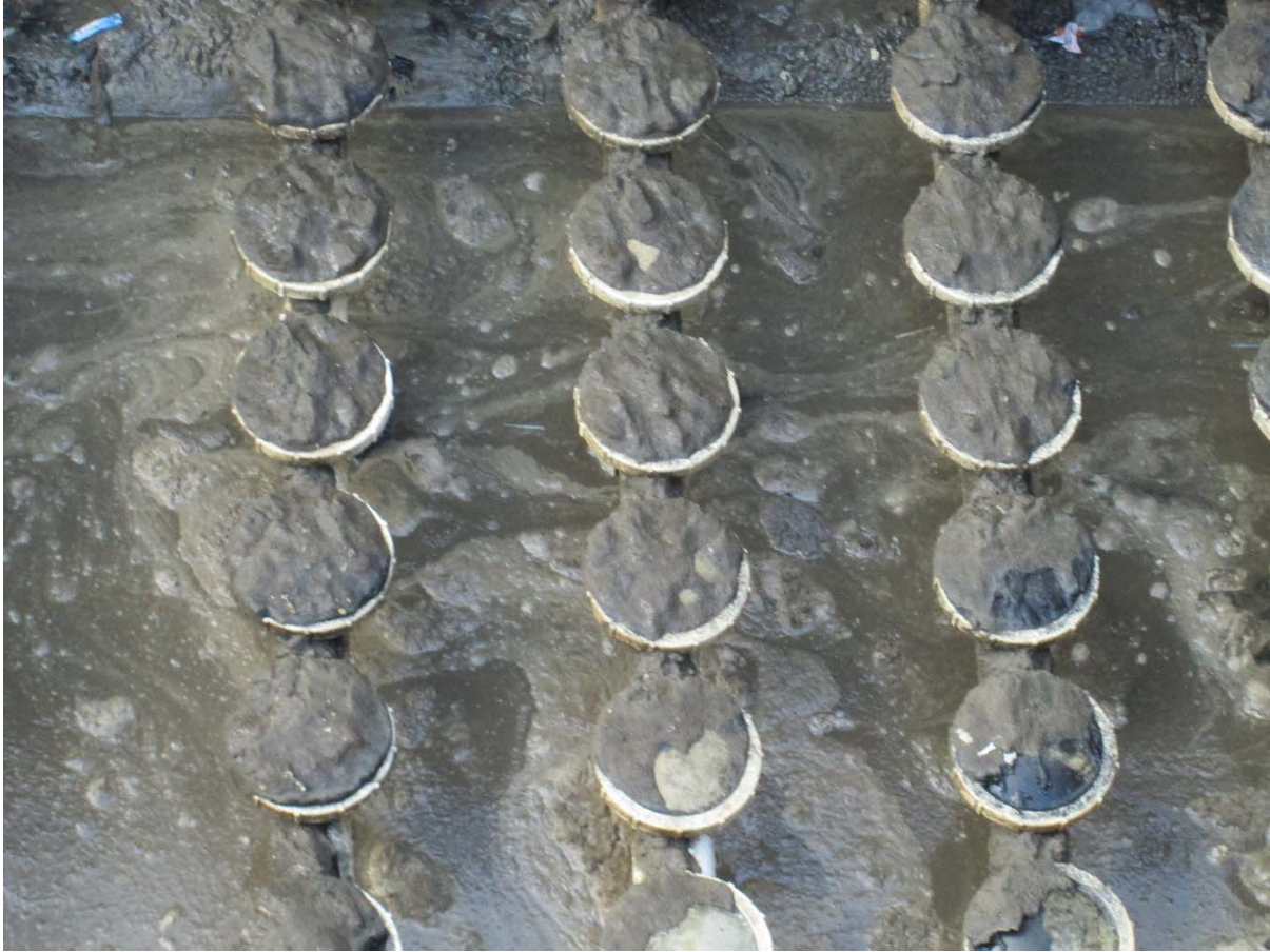
Figure 5: Settled sludge on membranes in anaerobic zones.
