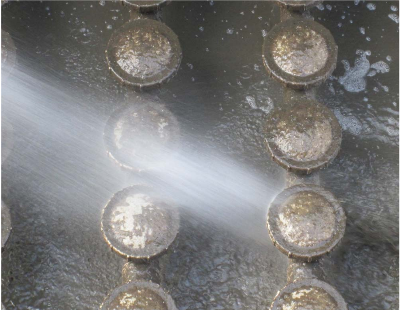
Figure 4: Membranes being sprayed to remove sludge film in aerobic zones.
