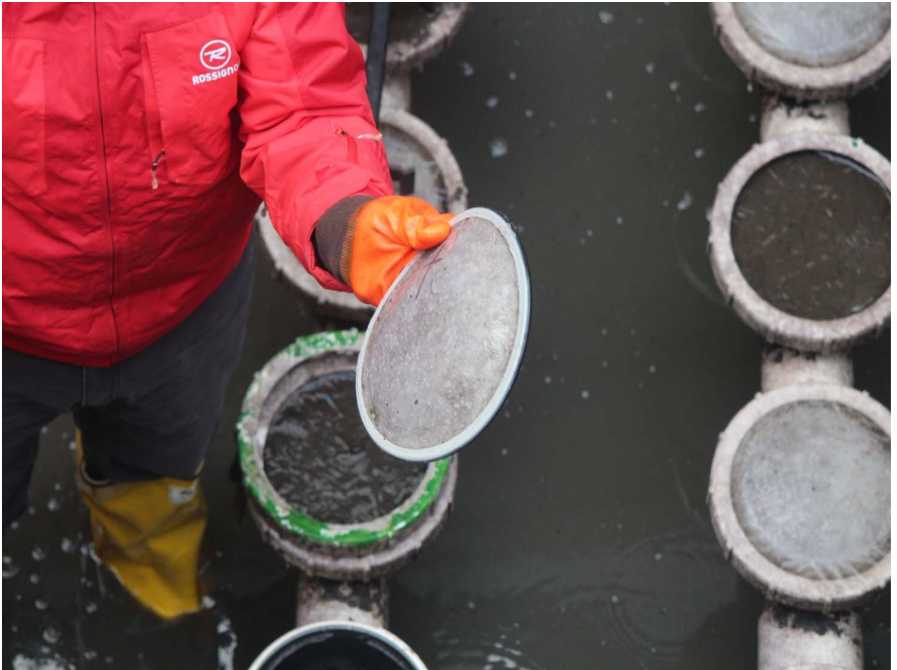
Figure 3: Marked membrane removed from base in aerobic zones for inspection and after spray washing
