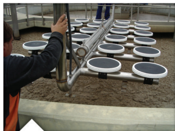
Disc diffusers provide exceptionally high oxygen transfer efficiency in this Spanish aeration tank
