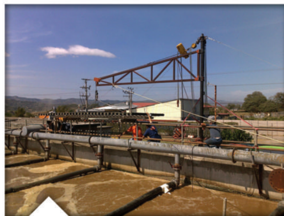
Retrievable grid with SSI Snappy Saddle Diffusers and a 304 SS frame replacing an underperforming floating lateral system
